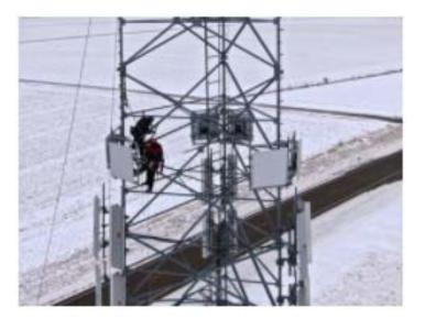
116. On information and belief, by locating the base station away from an area, and then transmitting the signal horizontally toward the area using antenna array panels facing the horizon, the Gogo 5G base station antenna array defines "a first radiation pattern focusing energy toward the horizon," as recited in claim 1 of the '077 Patent.
