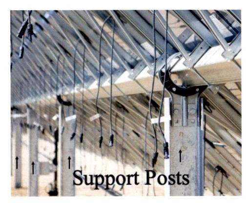
61. Defendant uses solar trackers that include a frame on which photovoltaic panels are mounted. The frame includes a torque tube beam which extends along the center of the frame. The torque tube beam is a central spine. The frame includes transversely arranged elongated members to which the photovoltaic panels are clipped. The elongated members are panel carriers.
