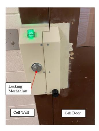
28. Habersham's Accused Product includes a first housing mounted to the exterior surface of said door with an opening in a side of the first housing that is adapted and arranged for receiving a lock bolt.
