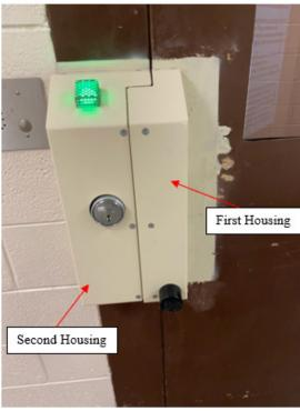
30. Habersham's Accused Product includes a strip protruding from the second housing and positioned substantially horizontally above and below the lock bolt for blocking access to the lock bolt and located between the first housing and second housing.
