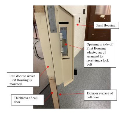
29. Habersham's Accused Product includes a second housing enclosing a lock for actuating a lock bolt adapted and arranged for being received by the opening in the side of the first housing adjacent to the lock bolt when the door is closed.
