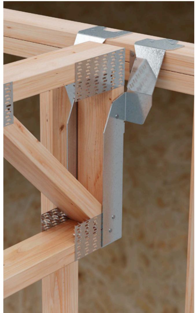
DGHT fire wall hanger installation.
