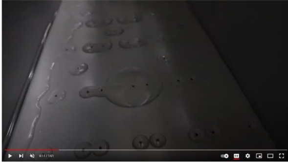
Riot Blockchain's 700 MW Bitcoin Mining Facility - 200MW Industrial-scale Immersion System
