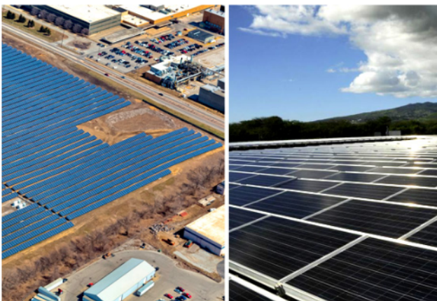
10.86-MW Maywood Solar Farm in Indianapolis (Left) and 5-MW Kalaeloa Renewable Energy Park in Hawaii, U.S.A. (Right)
