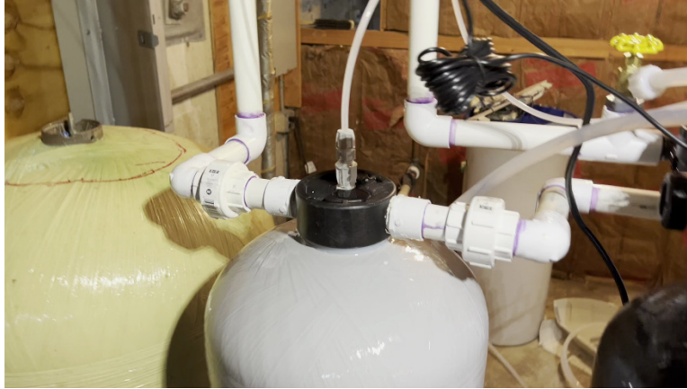
Figure 6: Another Image of the Infringing System
