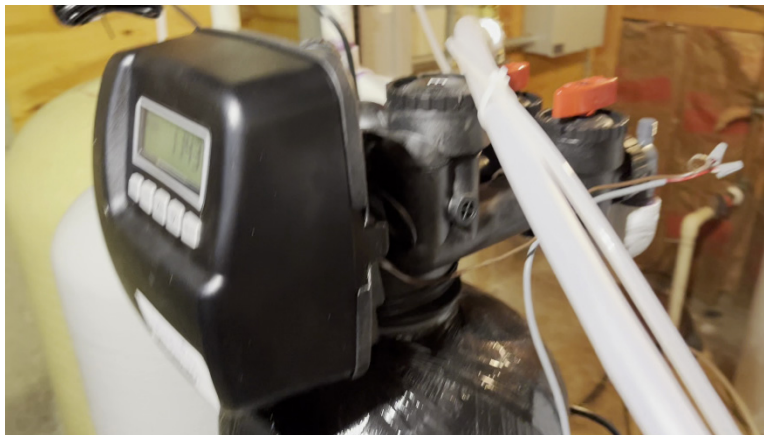
Figure 5: Another Image of the Infringing System
